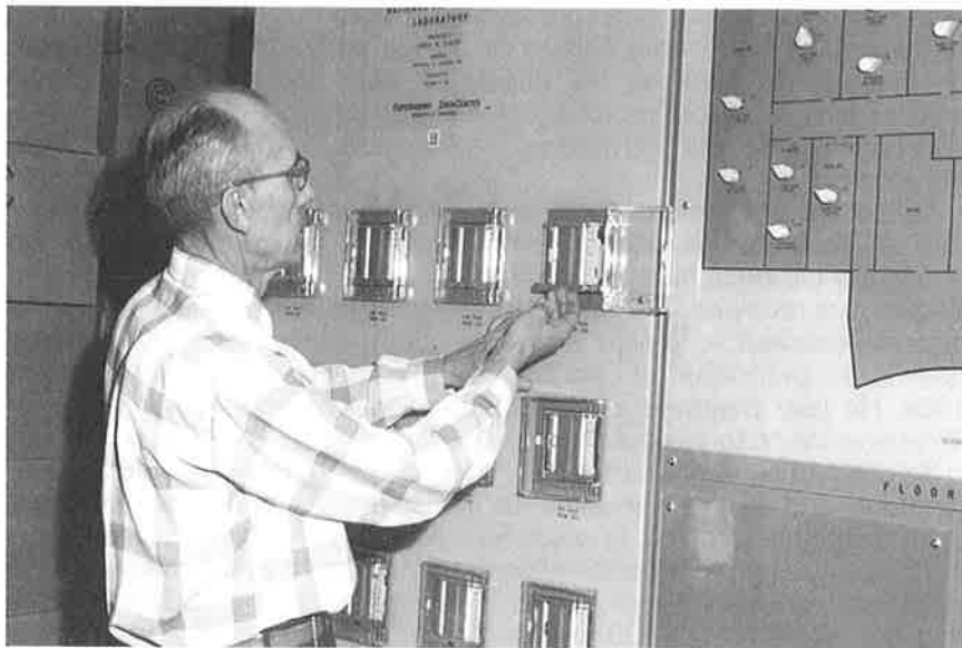
Figure 3. Dr. Edwin James checking the control panel for the seed storage vaults. Initially the storage vaults were maintained at 5°C and 40% relative humidity. The difficulties in maintaining RH and the storage studies conducted by Drs. Bass and James eventually led to lowering the storage temperature to -18°C and drying the seed before sealing in moisture proof bags, thus eliminating the need to control RH.
